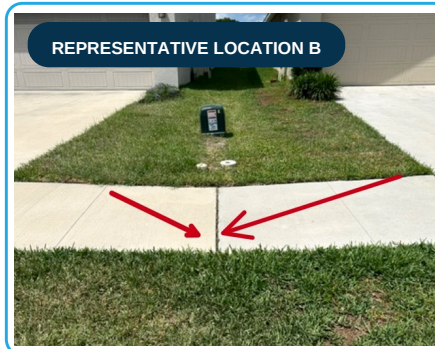
Matching settlement condition at second representative location.
